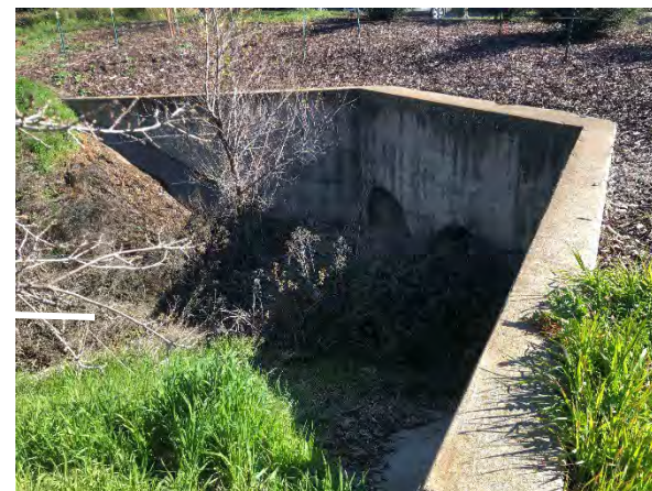
Blackberry blocking culvert inlet at downstream end of Mitigation Area B
