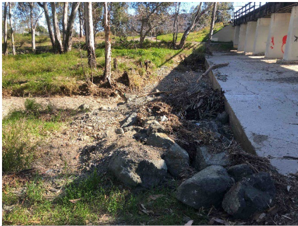
Scour pool below concrete of old railroad bridge, looking east
