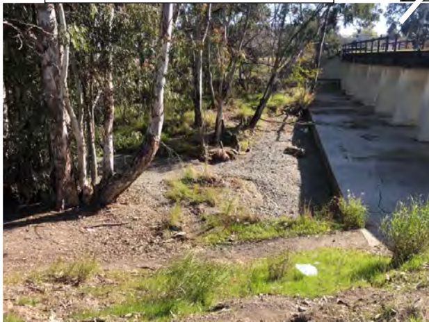
Concrete apron and scour pool
