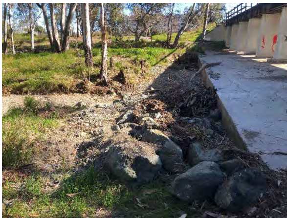
Scour pool below concrete of old railroad bridge, looking east
