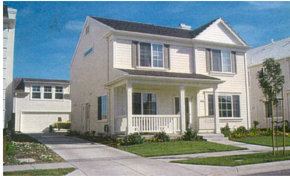
Detached garage (with habitable space above)
