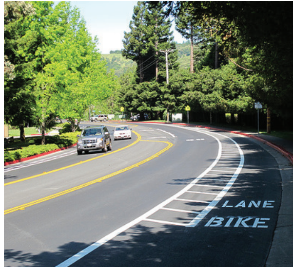
The use of pavement markings delineates space for cyclists to ride in a comfortable facility.
