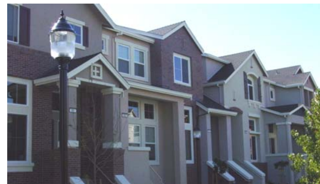
Roof designed as part of the building.
