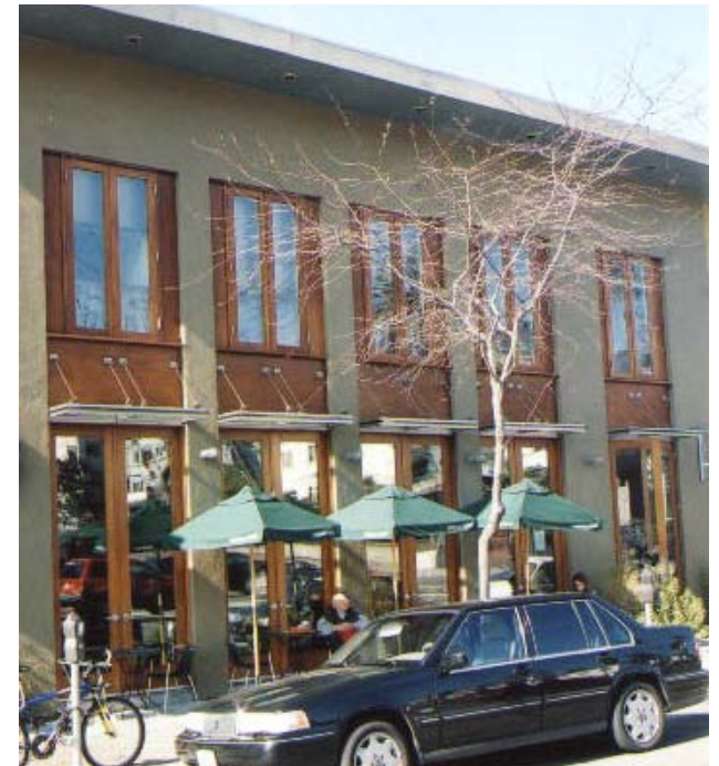
Upper floor windows should be smaller than storefront windows on the ground floor.
