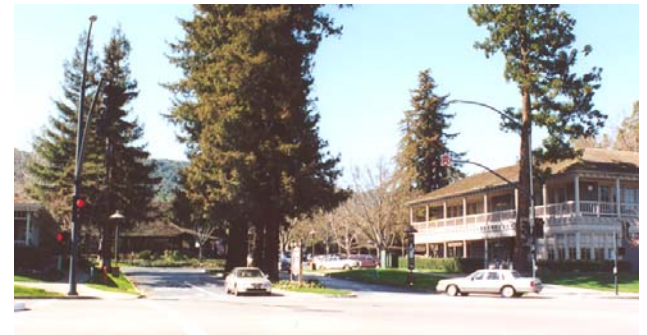
Existing redwood trees were incorporated into parking access alignment.
