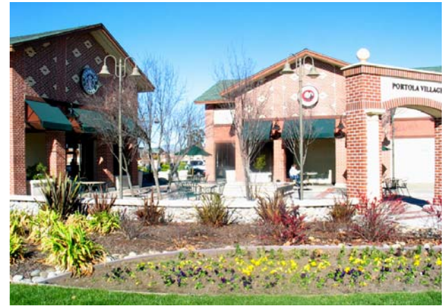
Street corner designed with public plaza.
