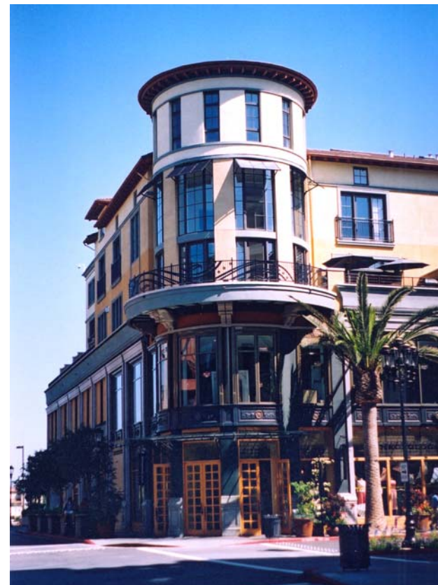
Taller building mass enhances the corner of a prominent location.
