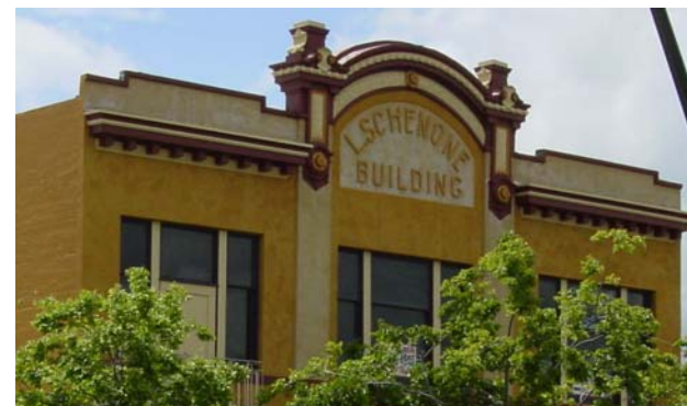
Shaped parapet with edge definition reflects overall building design.
