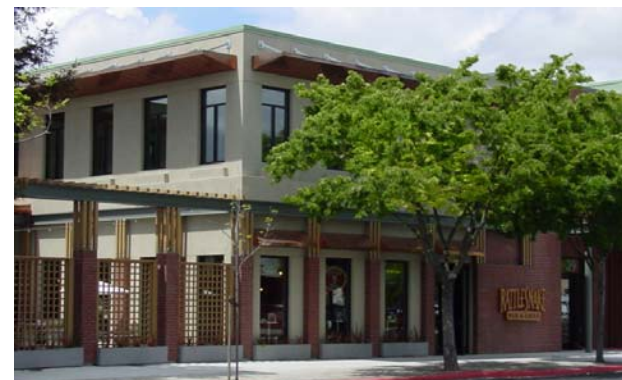
Canopies and recessed window bays help define the top and base of the building.
