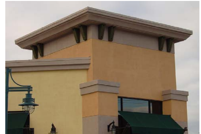
Flat roof with overhang.
