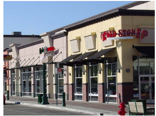
Harmonious window pattern throughout street frontages.
