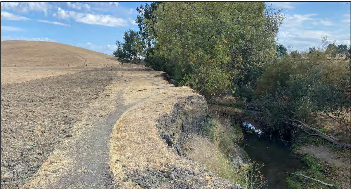
Photograph 8. Photo taken October 7, 2021 facing east. View of deeply incised top of bank within Arroyo Seco and scattered willow riparian vegetation.
