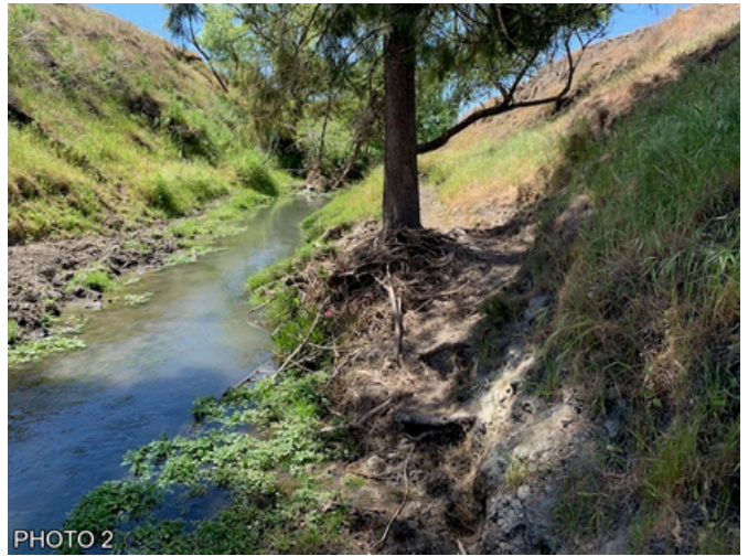
UPSTREAM OF PROPOSED SANITARY SEWER
