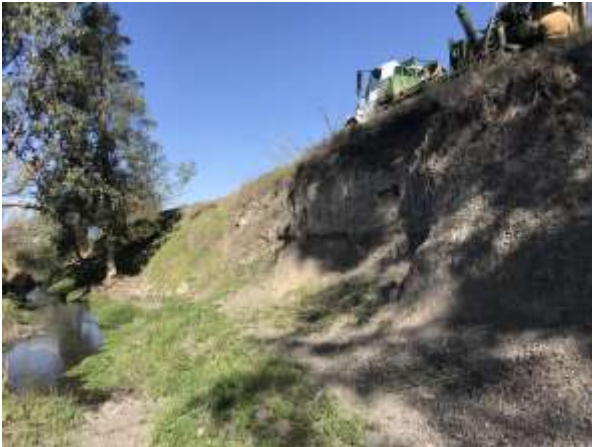
PHOTO 2.7-3: Shallow Sloughing of Southern Bank West of Proposed Bridge and East of Revetment Associated with Abandoned Bridge
