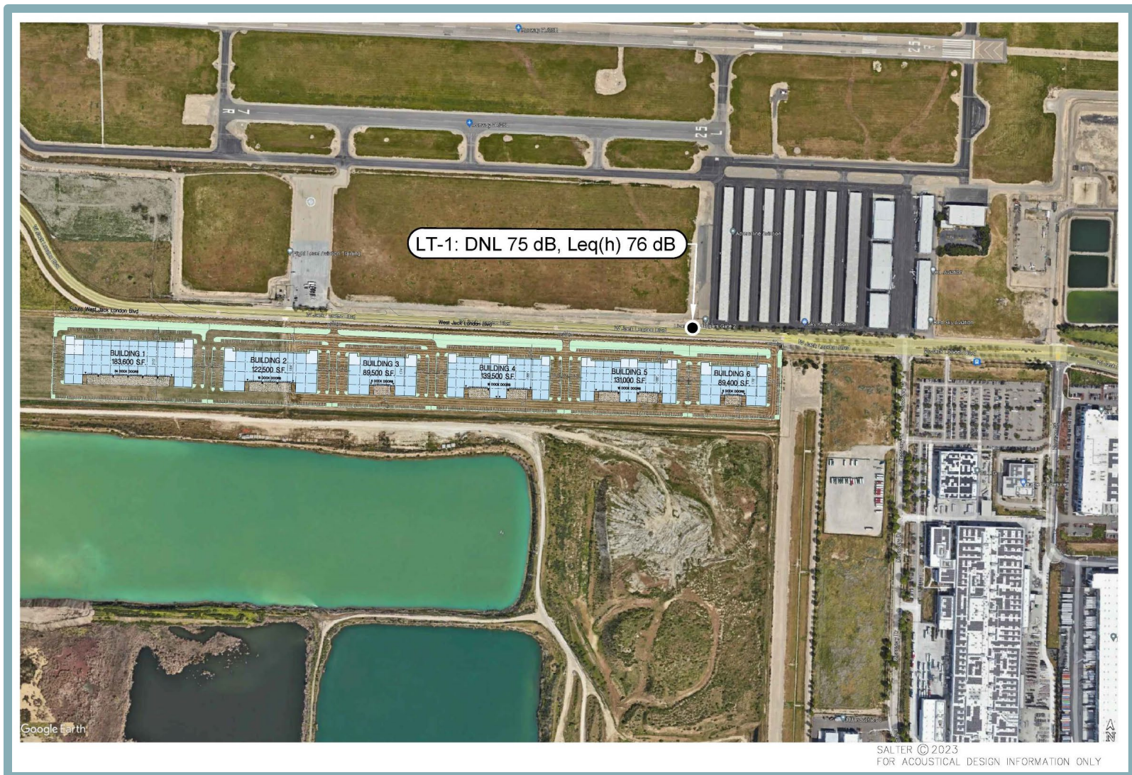
Figure 4.6-1 SMP 39 Ambient Noise Measurement Location
