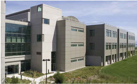
Developing modern office buildings will make Livermore a competitive place for innovative companies.
