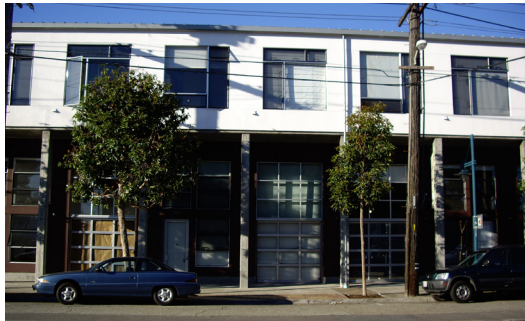
Developing a range of housing options, including multi-family housing (above) and live-work units (below) will provide a greater range of housing types for people in the region.
