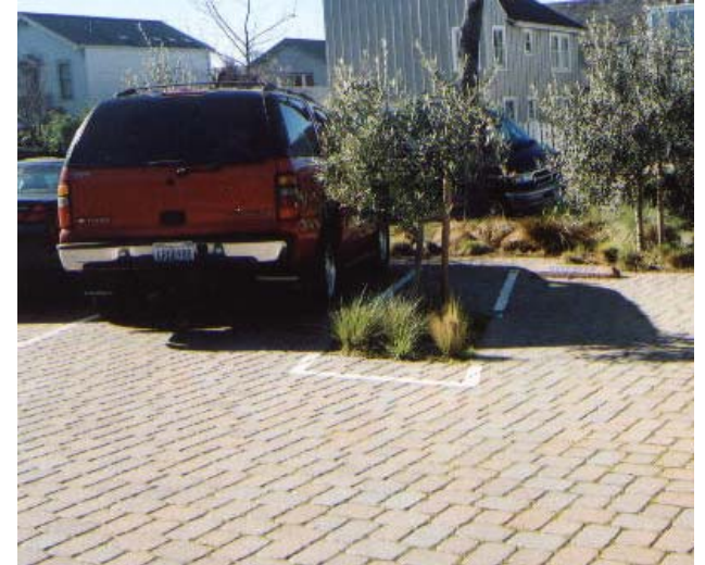
Water drains through permeable surface material into the ground.
