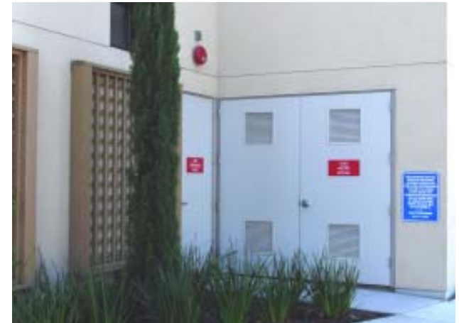
Utilities enclosed in building.
