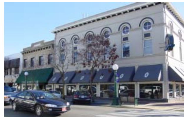
Awnings fit to the horizontal components of the ground floor building structure.
