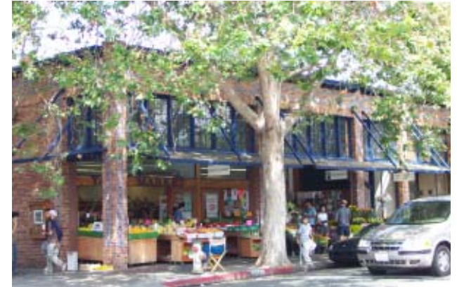
Individual tenants operate from separate structural bays of the building.
