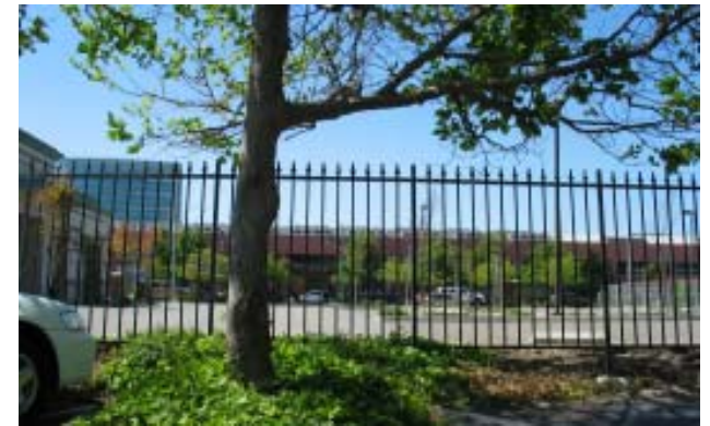
Unobtrusive fence design contributes to overall building and site design.
