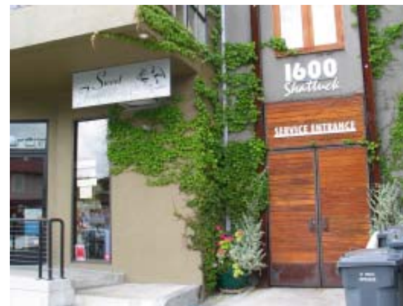
Service entrance clearly signed with materials consistent with other building components.
